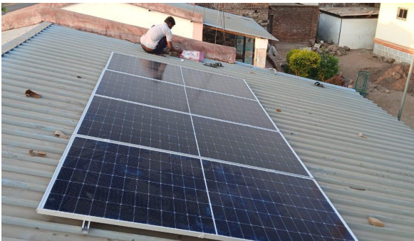
Solar Panels installed at Askhed
