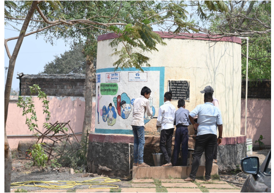
Low Flow Taps Installation, Koye
